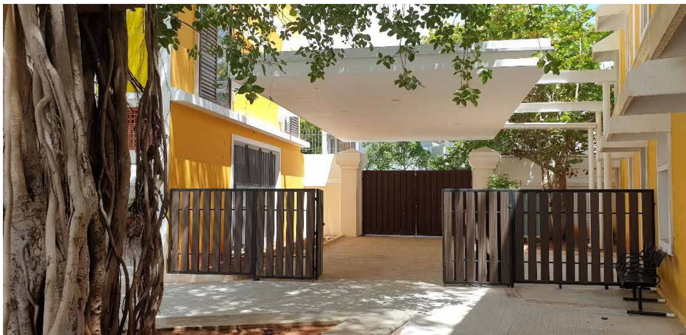
Entrance canopy suspended between the old and the new.
